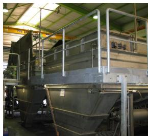
The fatty sewage from the production of a metal processing company is purified continuously by the addition of precipitation and flocculation agents and subsequent separation of ingredients in a flotation plant (< 250 m<sup>3</sup>/h). The optimal dosage of chemicals and control of the discharge is fully automated by **ARU** dosing control systems.
