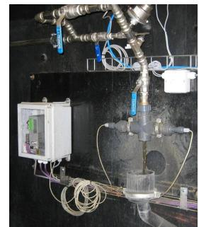
The clear water outlet of the flotation plant is also monitored by a contactless **ARU** transmitted light measurement.
