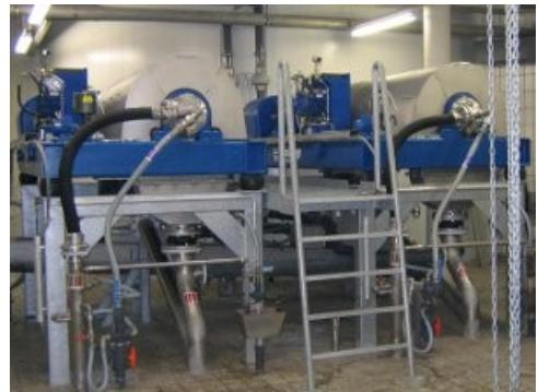
Objective of the measure is a consistently good dry matter content in the sludge discharge, a consistently good quality of the centrate and their continuous monitoring.
