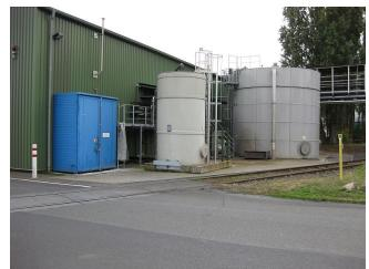
The dosage of both chemicals originally took place in continuous-flow stirred vessels. The vessels were replaced by a reaction line with some elbows. The amount of chemicals is now controlled by **ARU** dosing control systems and **ARU** - transmitted-light measurements.
